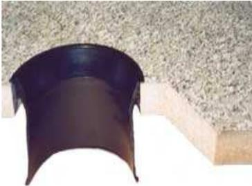
5) Make a pressure on top of the collar ring until the glue dries up. (Consult manufacturer recommendations for the time required)
