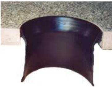
6) In materials as stone, marble, corian you can use a single plier to break the collar ring around the wastebin and then file or sand before to glue the wastebin.
